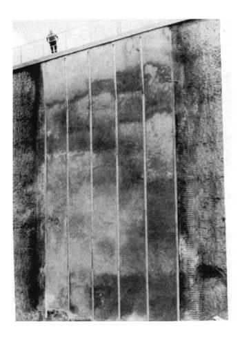
Figure 8-61. Steel profiles embedded in shotcrete, Cignana Dam
