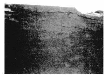
Figure 2-10. Parallel individual cracking caused by freezing and thawing
