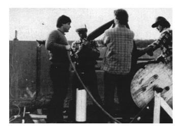
Figure 8-23. Two-component natural rubber and elastomer coated nylon sleeve being inserted into drill hole, Bagnell Dam
