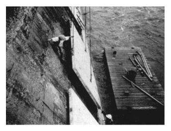
Figure 8-17. Installing precast concrete panels used to overlay the back side of the river wall at Troy Lock, Hudson River (Miles 1993)
