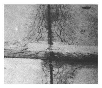
Figure 2-8. D-cracking in a concrete pavement
