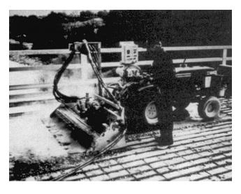
Figure 5-10. Hydromilling (water-jet blasting)
