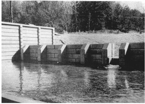
Figure 8-43. Precast concrete checkdams, Chauncy Run
