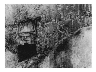
Figure 2-2. Honeycombing and cold joint
