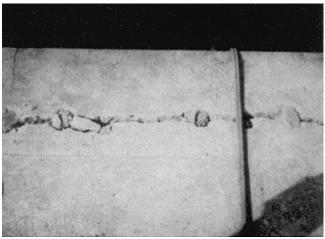
Figure 5-12. Presplitting using chemical-expansive agent
