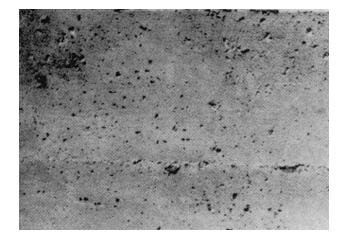
Figure 2-1. Bug holes in a vertical wall
