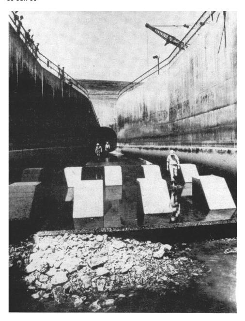
Figure 8-30. Stilling basin dewatered for inspection, Pomona Dam
