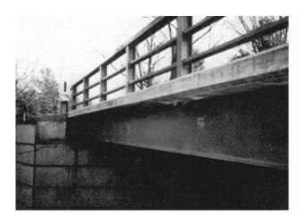
Figure 8-53. Precast abutment and deck units, Ulsterville Bridge
