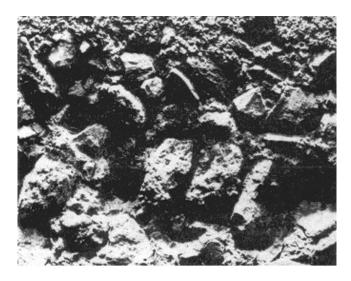
Figure 2-21. Rough, pitted concrete surface caused by cavitation
