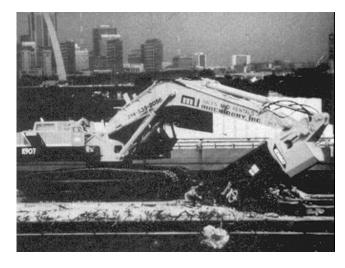
Figure 5-2. Boom-mounted concrete crusher
