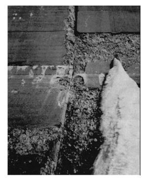
Figure 2-19. Very severe scaling
