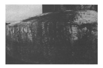
Figure 2-7. Pattern cracking caused by alkalicarbonate reaction
