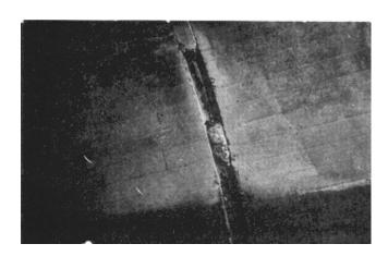
Figure 2-22. Deterioration of joint sealant
