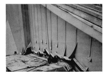
Figure 8-62. Installation of geocomposite, Pracana Dam
