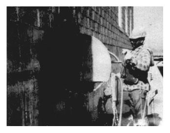
Figure 5-3. Diamond-blade saw
