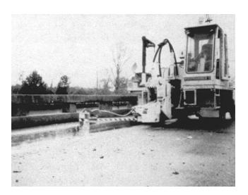
Figure 5-8. Spring-action hammer (mechanical sledgehammer)
