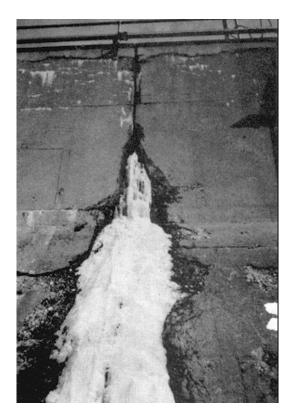
Figure 2-28. Water seepage through joint
