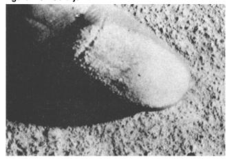
Figure 2-4. Dusting on horizontal finished surface
