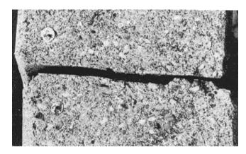
Figure 2-23. Loss of joint sealant
