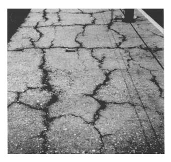
Figure 2-6. Pattern cracking resulting from alkali-slice reaction
