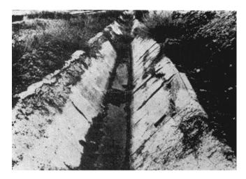
Figure 2-14. Disintegration of concrete caused by sulfate attack
