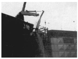
Figure 5-11. Rotary-head milling
