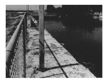
Figure 2-18. Severe scaling
