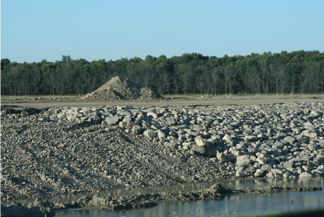
Figure 7.3.7.2-1. Riprap and bedding in construction.
