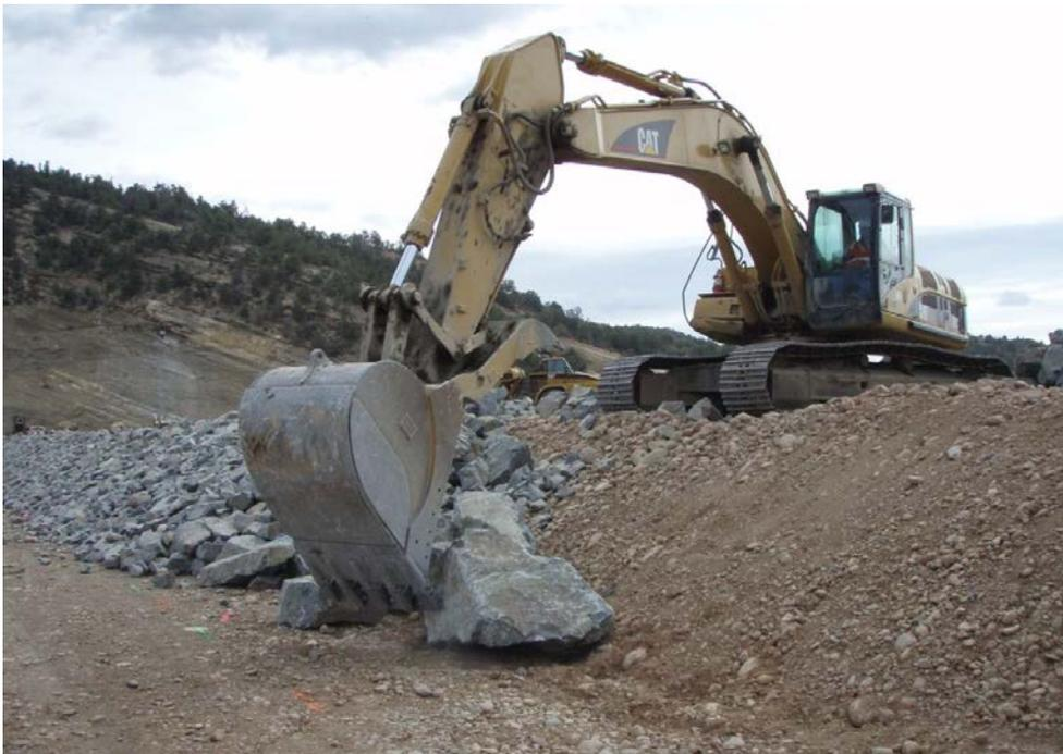
Figure 7.4-1. Careful placement of riprap (note the small drop height).
