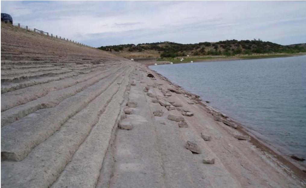
**Figure 7.5-1. Typical aged soil-cement slope protection.**
