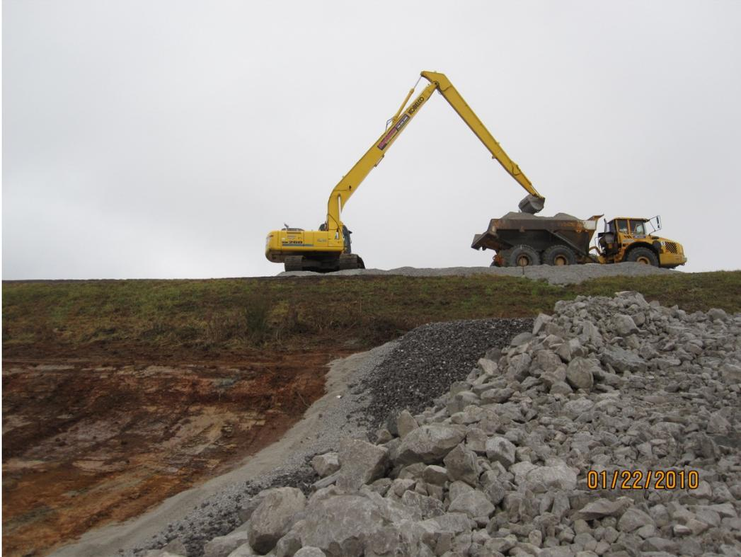
Figure 7.3.7.5-2. Photo presenting use of two bedding layers.
