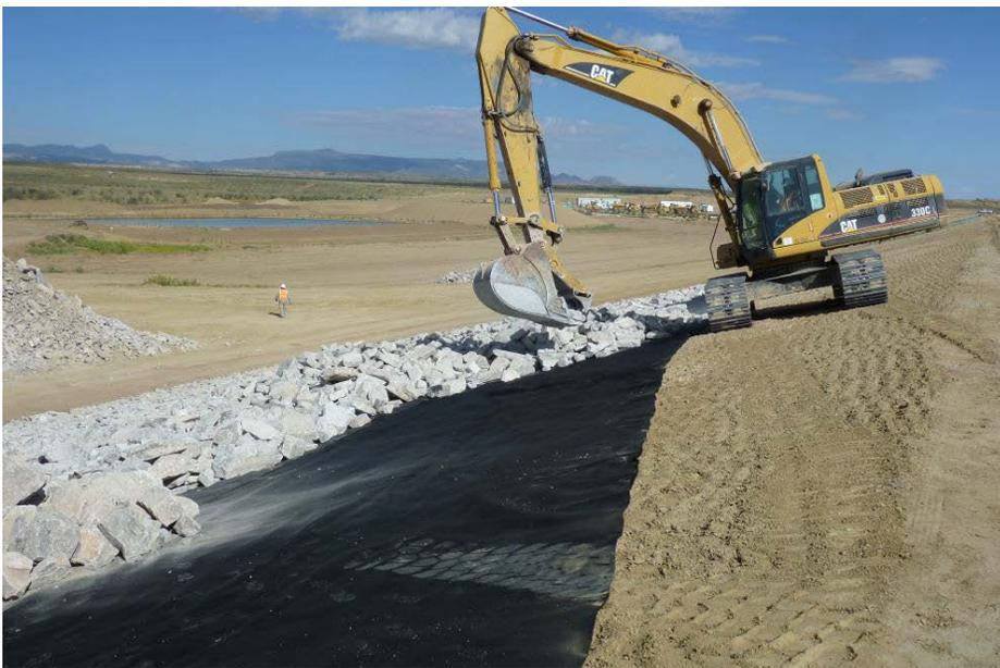
**Figure 7.5-3. Riprap being placed on a geotextile serving as bedding.**
