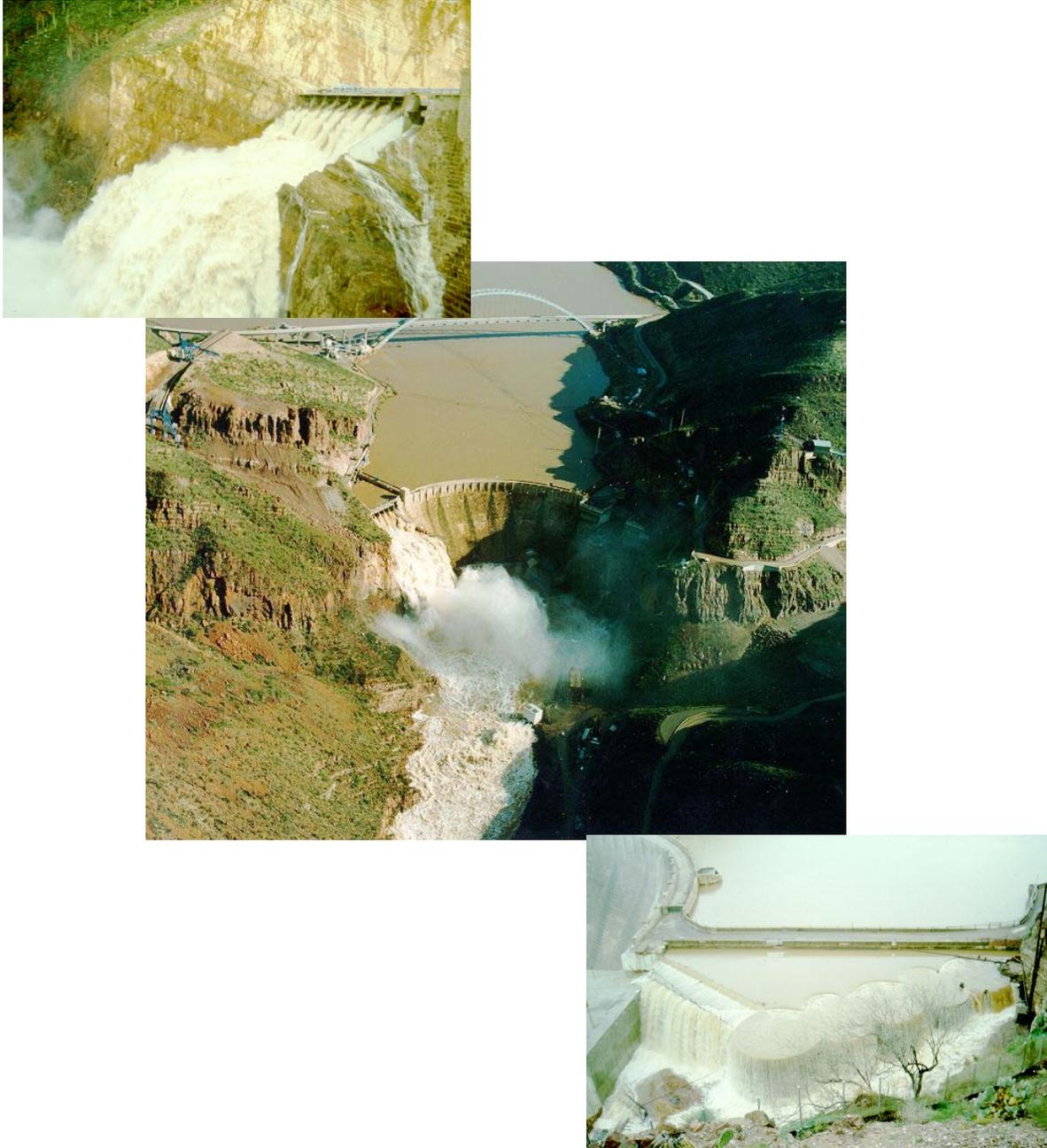
**Figure 2.2.1-1. Example: Flood event (estimated inflow peak of about 89,600 cubic feet per second [ft<sup>3</sup>/s]) occurred during construction of a dam safety modification in 1993 (center photograph). This resulted in the existing right abutment service spillway passing about 41,600 ft<sup>3</sup>/s (upper left photograph), and the left abutment cellular cofferdam being overtopped, but failure did not occur (lower right photograph). Theodore Roosevelt Dam, Arizona.**
