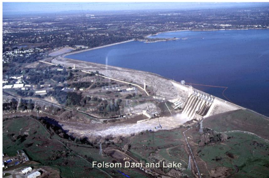
**Figure 2.2.1-3. Example: Flood event (estimated inflow peak of about 298,000 ft<sup>3</sup>/s) occurred in 1997. This was one of many significant floods resulting from a weather phenomenon referred to as the “pineapple express.” Folsom Dam, California.**
