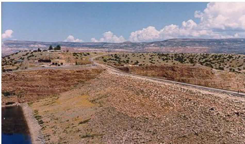
**Figure F-3. Example 3: additional fill to raise the embankment**
