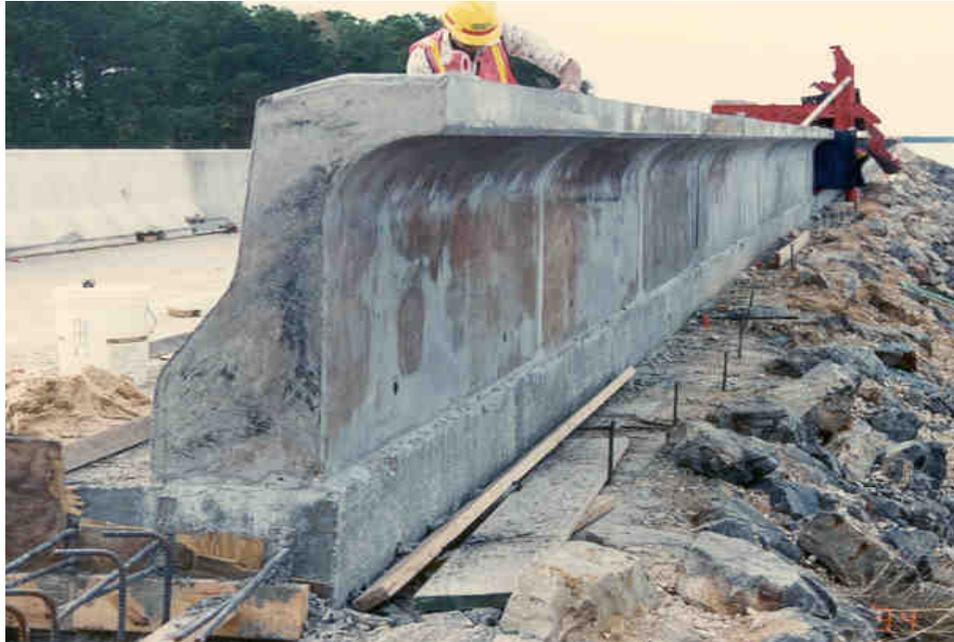
Figure F-1. Example 1: curved parapet wall, maximum protection against wave action
