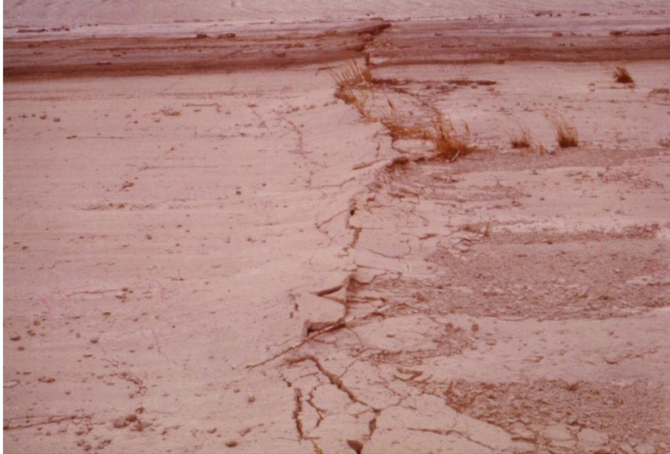
**Figure 17.5.5-3. Damaged soil-cement slope protection on the 10H:1V beaching slope at Merritt Dam, Nebraska.**
