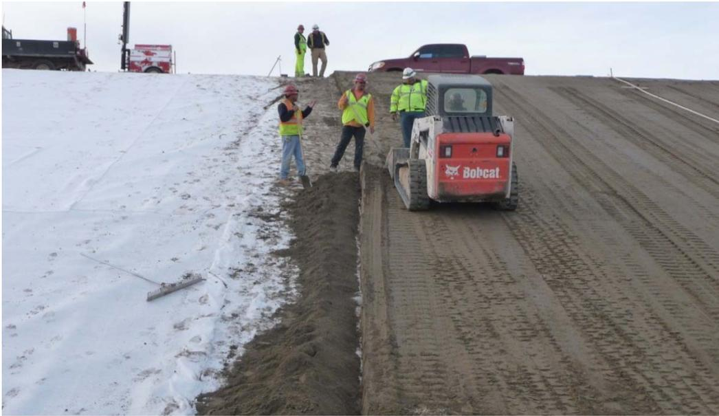
Figure 17.6.5-1. Trimmed vertical construction joint at Warren H. Brock Reservoir, California.
