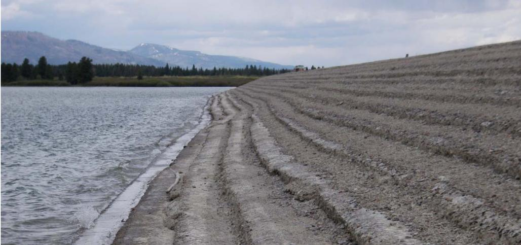
Figure 17.4.2.2.3-1. Soil-cement slope protection at Jackson Lake Dam, Wyoming.
