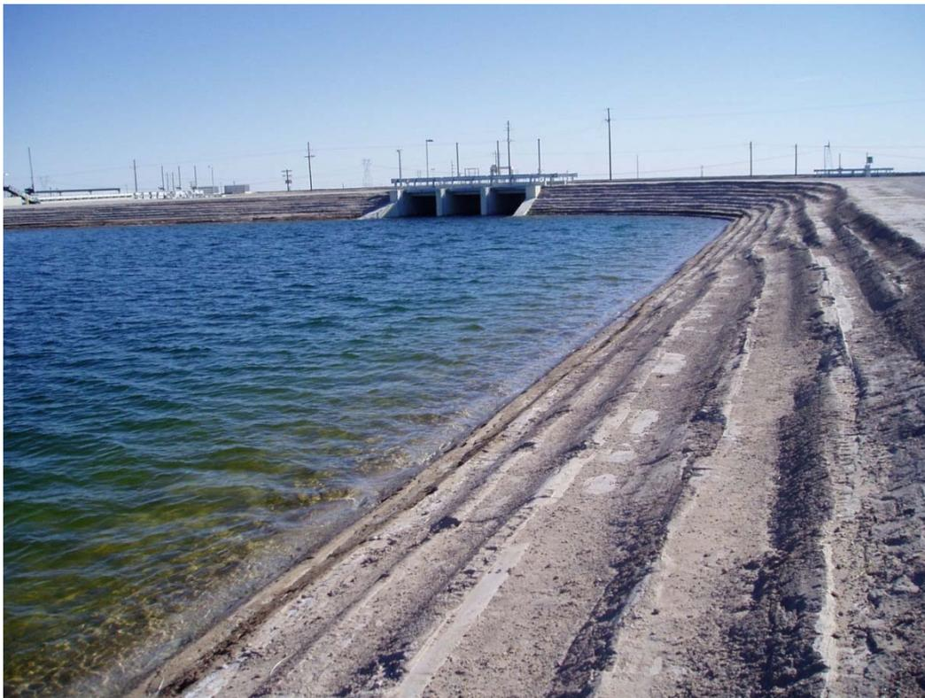
Figure 17.5.3-2. Stairstep soil-cement at Warren H. Brock Reservoir, California.
