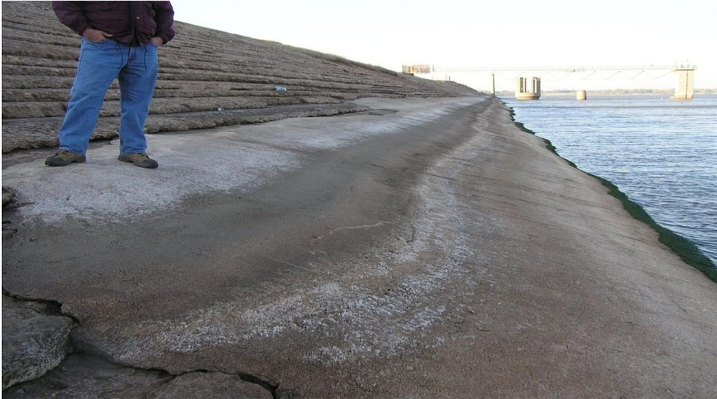
**Figure 17.2.2-4. Closeup view of concrete patch on soil-cement slope protection at Cheney Dam, Kansas.**
