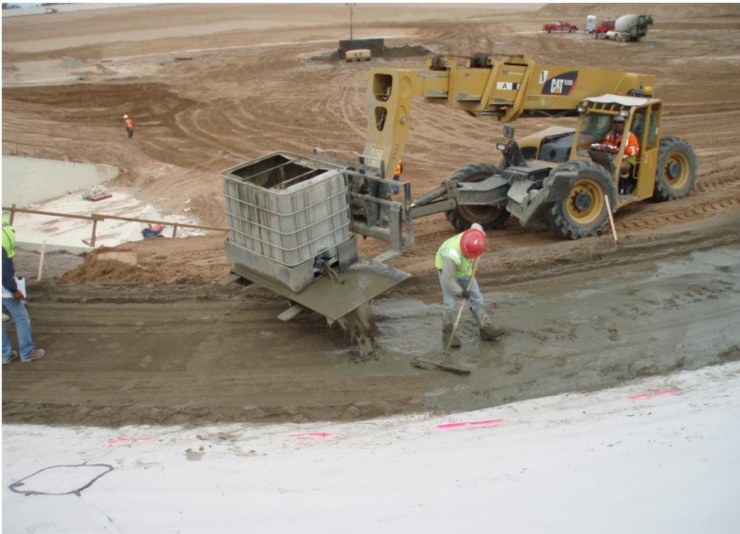
**Figure 17.5.7-1. Spreading of cement slurry bonding agent at Warren H. Brock Reservoir, California.**
