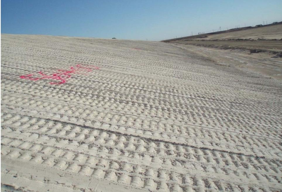
**Figure 17.5.3-3 Plating soil-cement at Warren H. Brock Reservoir, California.**
