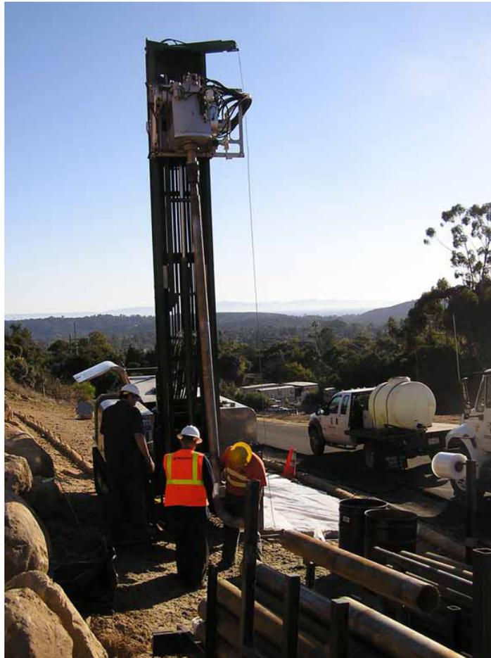
**Figure 12.8.8-1. Sonic drill rig. The sonic drill head works by sending high frequency resonant vibrations down the drill string to the drill bit.**
