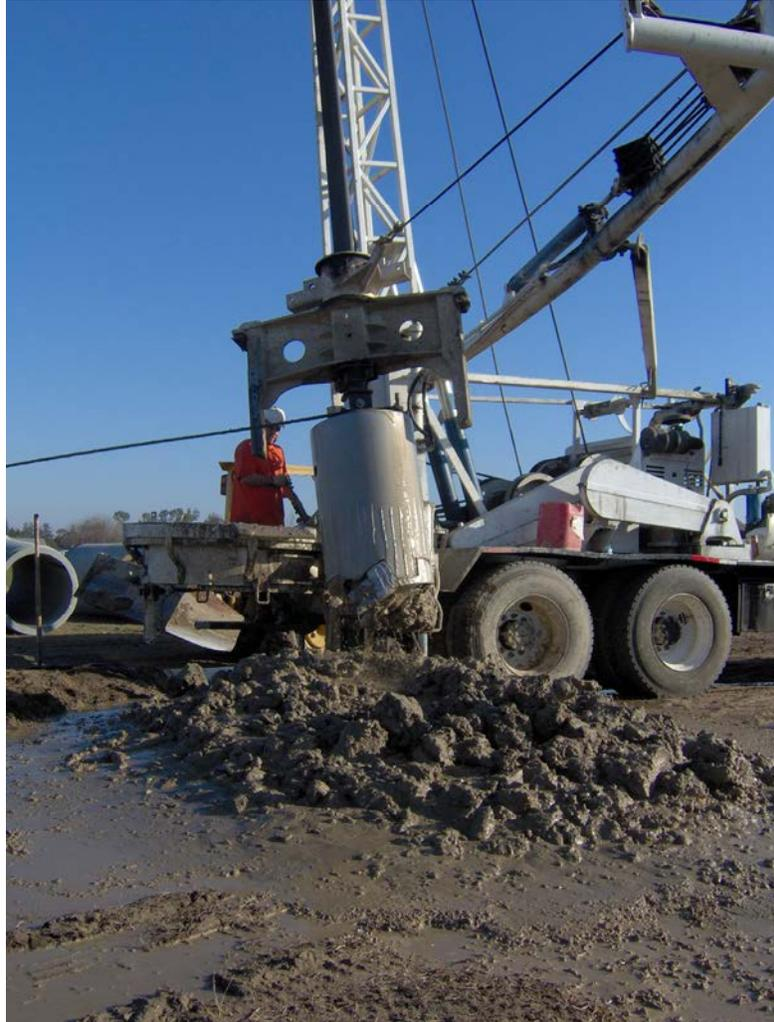
**Figure 12.8.2-3. Bucket auger being used with bentonite drilling mud.**
